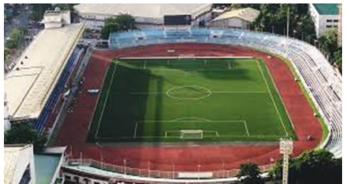
Philippines Sports Commission - Rizal Memorial Stadium Administration Building 2020 - Exit Signs, Fire Protection Signs, Evacuation Plans and Egress Path Marking Solutions
