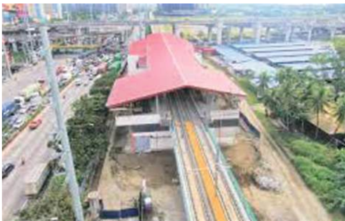
LRT-1 Cavite Extension - Redemptorist Station 2024 - Exit Signs, Fire Protection Signs and Egress Path Marking Solutions
