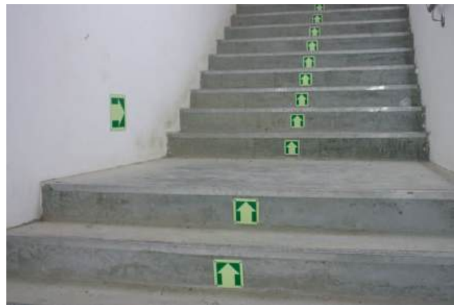
Marine Coastal Expressway - Singapore
