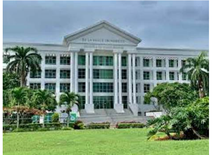
De La Salle University - Laguna Campus 2022 - Exit Signs and Fire Protection Signs
