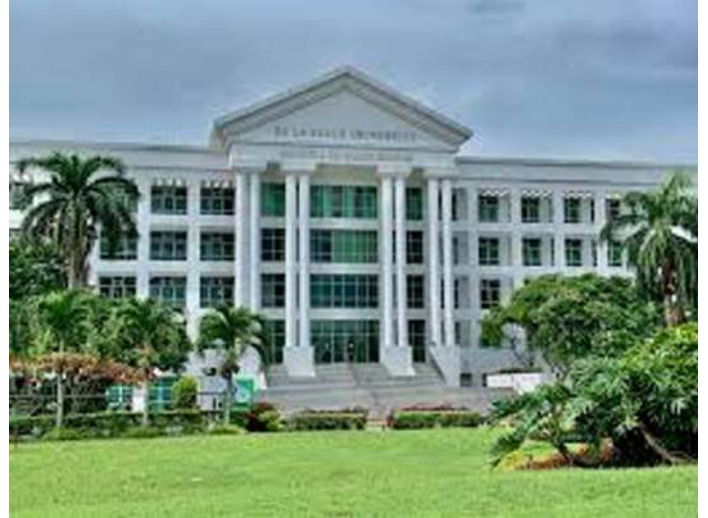
De La Salle University - Laguna Campus 2022 - Exit Signs and Fire Protection Signs
